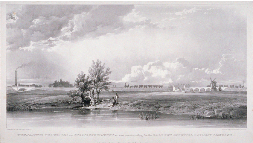
Figure 2. View of the River Lea Bridge and Stratford Viaduct as now constructing for the Eastern Counties Railway.
